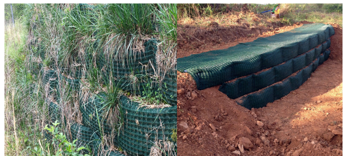
Figure 2 - Constructed and vegetated PYRAWALL
