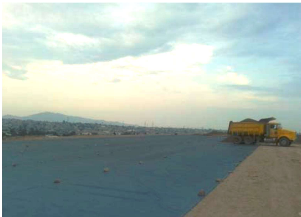
Image 1 - H2Ri Installed Parallel to Planned Traffic Flow Over a Prepared Subgrade
