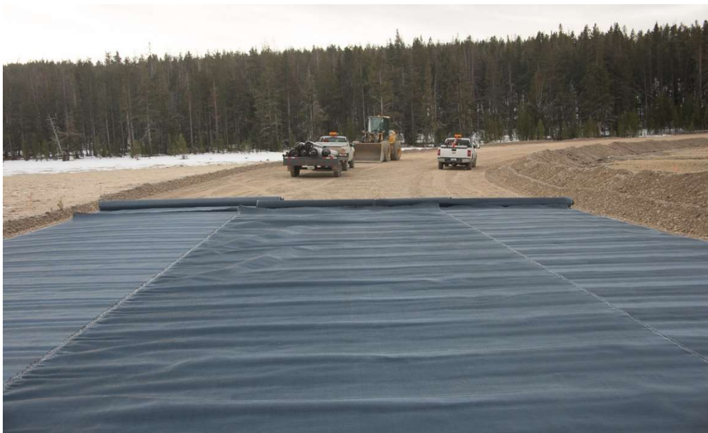
Image 3 - Center Roll at the High Point Moving Water to the Left and Right.
