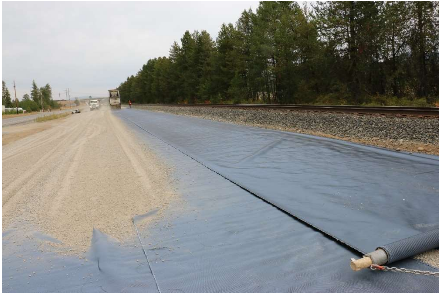
Image 16 - Forklift Pulling the Material Taut as Truck Begins its End Dump.
