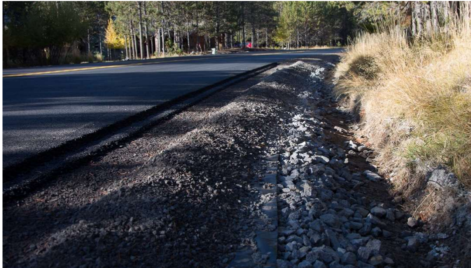
Image 8 - Edge Termination on Side of Embankment into Ditch Line (Right Side)
