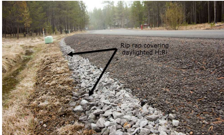
Image 9 - Daylighted Installation Using Rip Rap to Cover the Exposed Edge of Mirafi® H 2 Ri.
