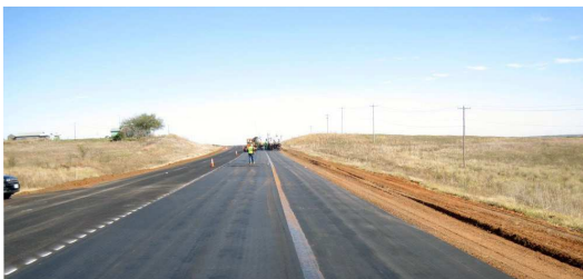
Image 3: All adjacent GlasPave should be overlapped.
