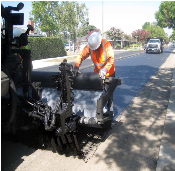
Image 2: Distributor truck with fabric applicator attached to the back.
