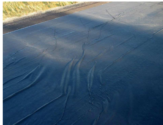
Image 5: Wrinkles after rolling that are 1 in. or greater should be slit and shingled in the direction of paving.
