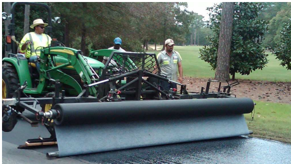
Image 1: Interlayer laydown equipment.
