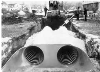
Multiple End Section on Round CSP
