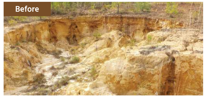
Large gullies formed due to erosion
