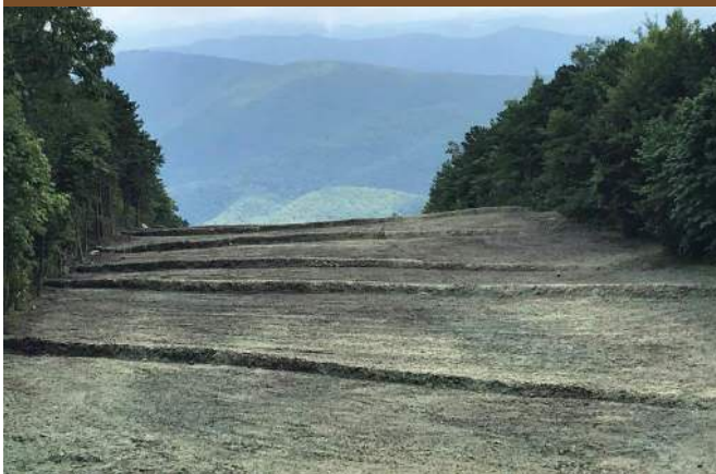
Energy / Pipeline Restoration
