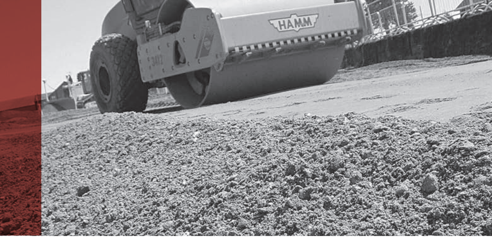
Compacting the aggregate fill.
