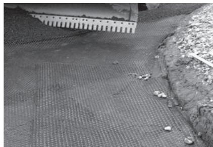
Placing Geogrid to accommodate curves.
