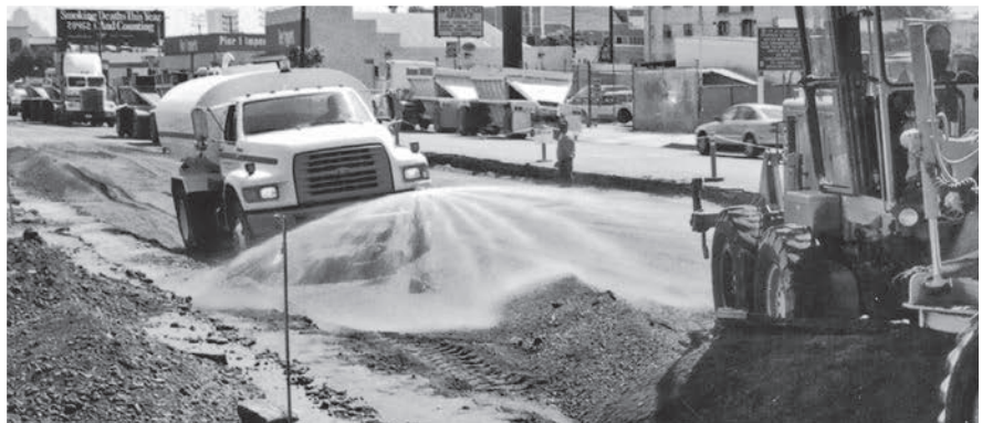
Moistening the fill before compaction.
