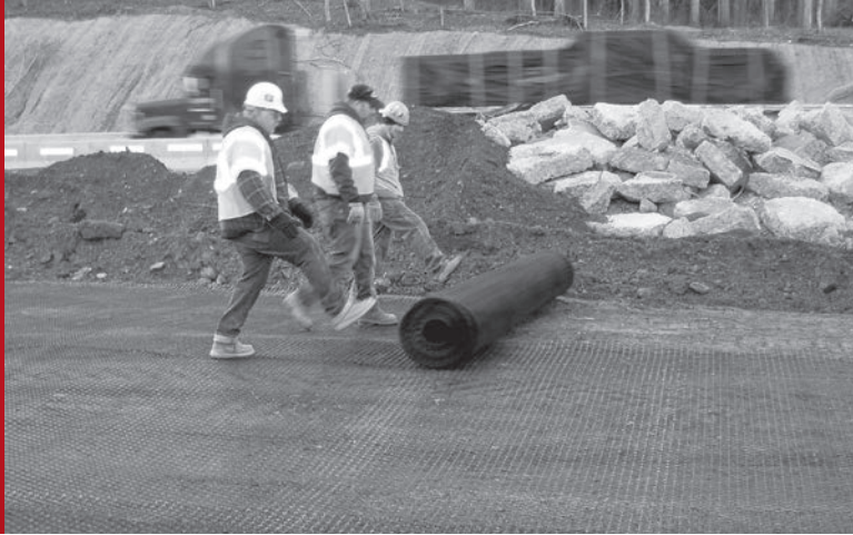
Rolling out Tensar® Geogrid.
