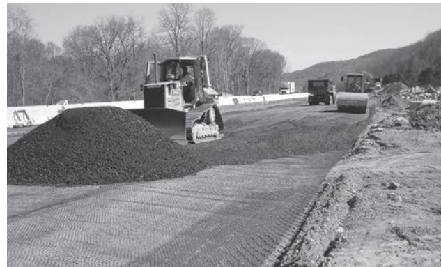
Spreading aggregate fill over Tensor Geogrid.
