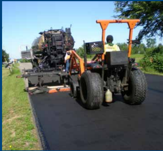
INSTALL FABRIC OVER LIQUID ASPHALT
